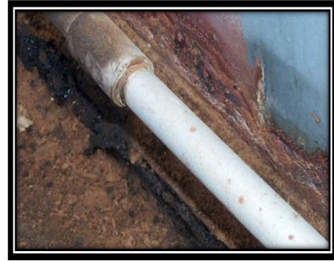
Fig. 2 The external side of the shell svere corosion
