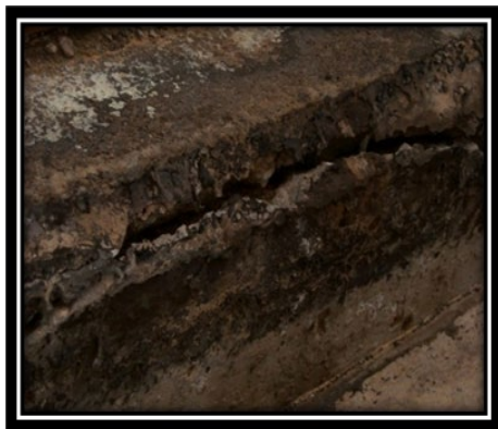
Fig. 1 Cracked concrete foundation ring of the tank.
