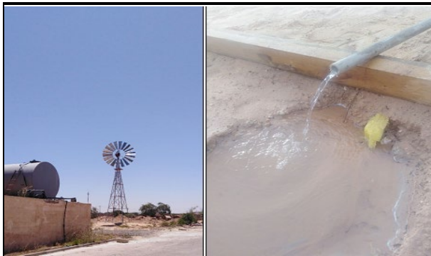
Figure 16. Extracting water from the Well by the Windmill system.
