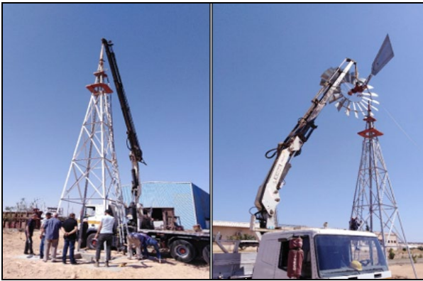
Figure 15. Rotor and tower installation.
